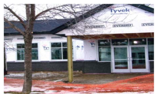
Pre-Siding Installation
