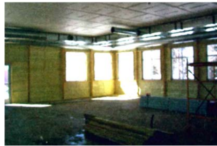
Window Installation & Insulation
