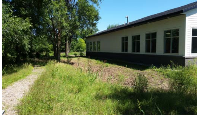
Back View of Final Stages (pre-landscaping)!
