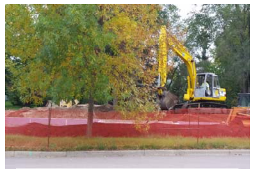
Excavating of Land
