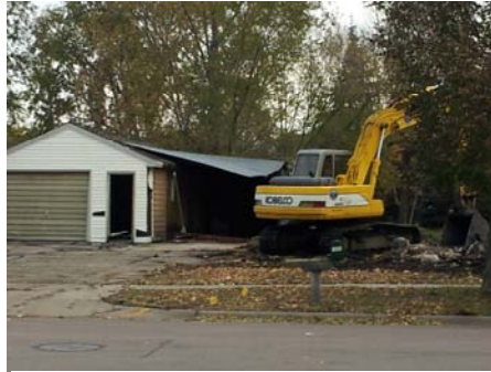
Bulldozing of Existing Garage
